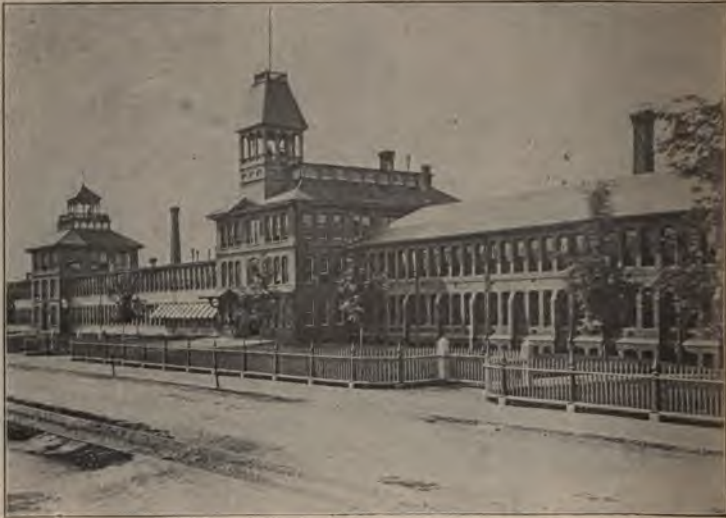
The Factory in 1870 from a Photograph.
