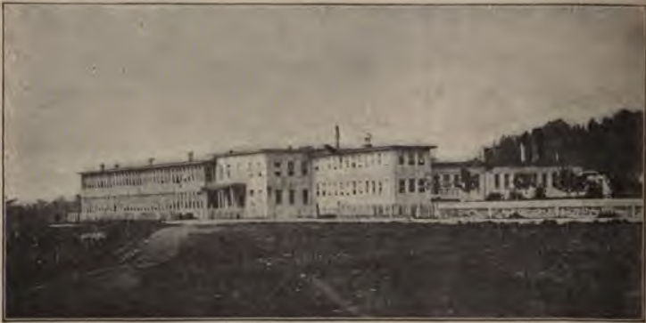
The Factory in 1863 from a Photograph.
