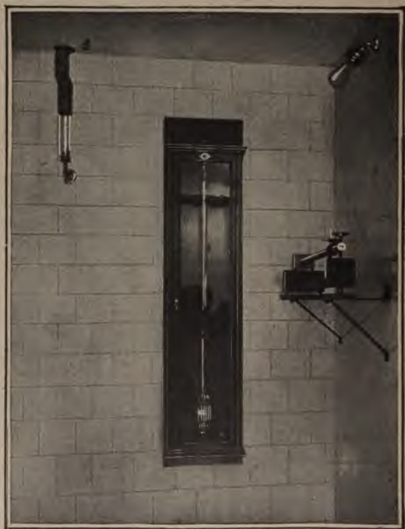
View in outer passage of Clockroom showing barometer and level tester.
