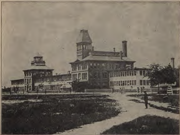
The Factory in 1865 from a Photograph.
